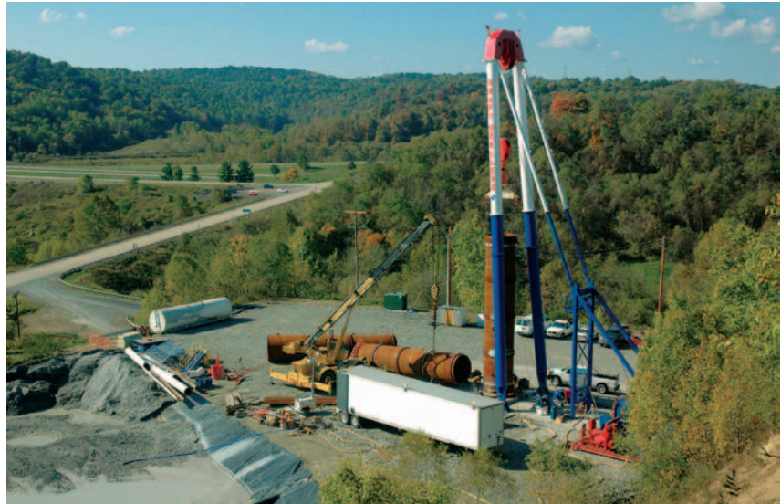
Shaft drilling operations are conducted from the surface with only a few miners.
